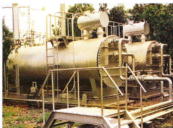
Heating Unit of RMS of 90 MW power station at Fenchuganj
